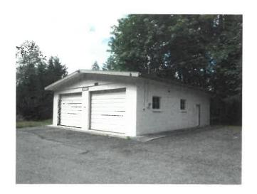
Fire Station 52, known as the Olympic View Community Fire Station, is one-story masonry structure, built on relatively flat ground. The 1963 building is rectangular in plan, measuring approximately 40 feet by 32 feet with an approximate roof height of 14 feet. Building construction consists of masonry walls supporting wood roof trusses. Fire Station 52 serves as a volunteer fire station for Central Kitsap Fire and Rescue and houses one engine.
