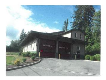
Fire Station 64, known as the Chico Community Fire Station, is a two-story wood and steel framed structure. The 1999 building is rectangular in plan at the first floor at 48 feet by 76 feet. The second floor of the building is primarily located on the west side with a small section also located at the center of the building; a small mezzanine is located between the two floors. Fire Station 64 houses one engine, one rescue vehicle, and one tender.
