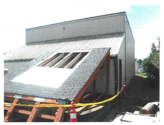
Figure 3.4-2. Fire Station 51 Maintenance Building, Roof Prop Leaning on North Exterior.
